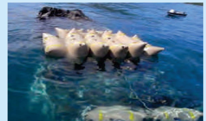
Shallow water wreck removal using clusters of Enclosed Flotation Bags 2,000 lbs.
